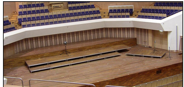
Figure 7: Stage with basic arrangement of stage risers. Height of stage: ~stringed instruments: 0 m (except basses: 0,25 m); ~wind instruments 1 st row: 0,25 m; ~wind instruments 2 nd row: 0,5 m; ~percussion: 1 m
