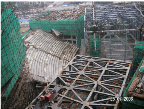
The theatre of CCTV under construction
